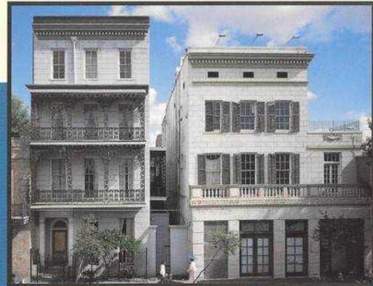
The same two buildings, 1993
